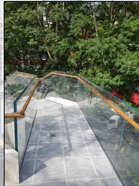
Glass Railings with Timber Handrail
