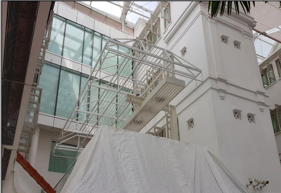
Painted Steel Canopy
